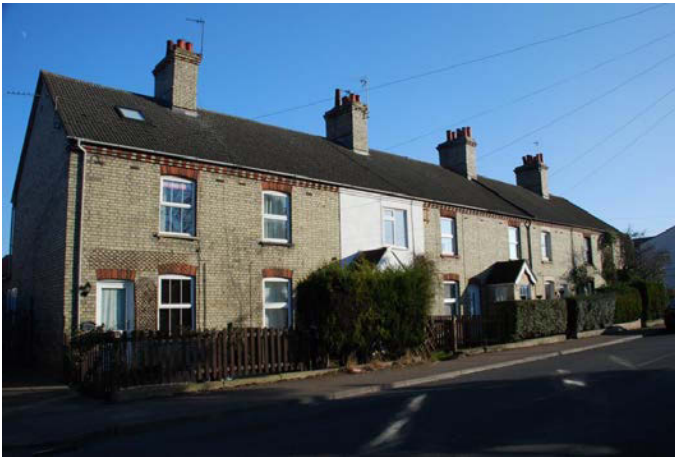
Example of characteristic cream brickwork
